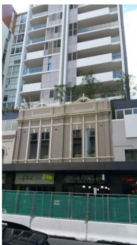
Facade retention at Bondi Junction retaining original street faced as an open frame.
